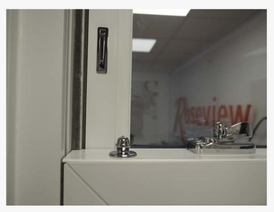
Normally the limit stops will be in the "out" position, which prevents the sashes from sliding more than around 100mm (4 inches)
