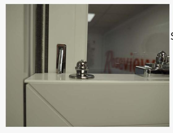
Your windows may be fitted with limit stops (called "shark fins"), which restrict the amount that the top and bottom sashes can open to around 100mm (4 inches). These can be temporarily closed to allow your windows to open more.
